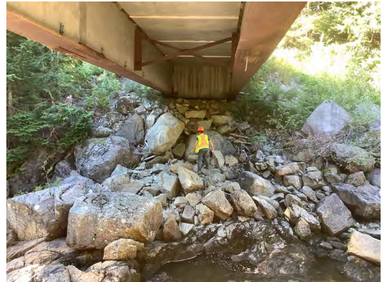
Right Bank Abutment when facing downstream
