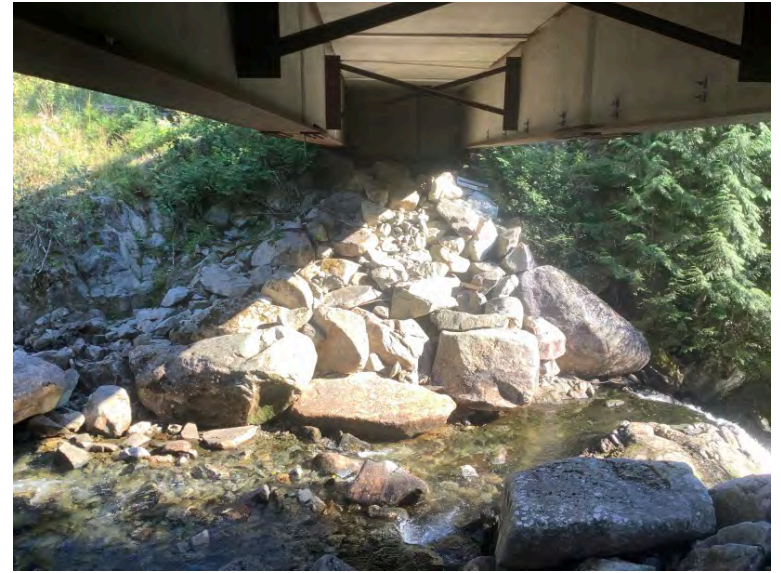
Left Bank Abutment when facing downstream
