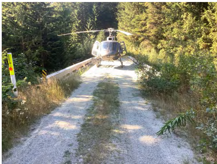
Approach from Left Bank when facing downstream
